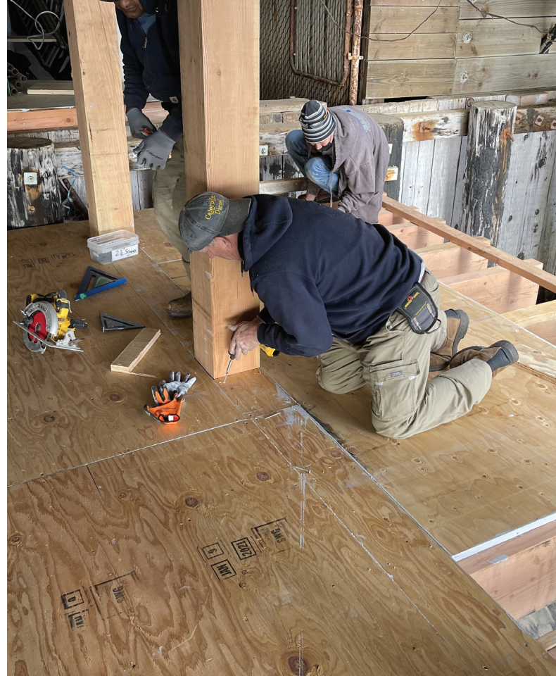
NEW COATINGS Workers repair beams under coastal homes.
